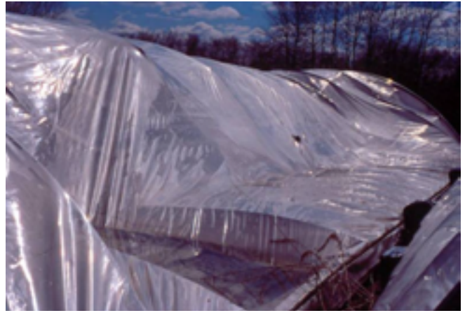
Greenhouse collapsed by snow load
